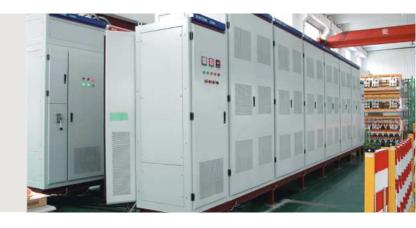
The STATCOM device consists of five parts: control cabinet, power cabinet, start panel, connection reactor and power transformer.
